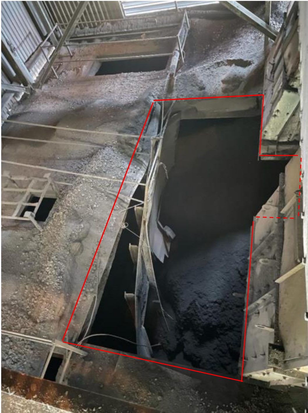
Figure 1: Outline Damaged Platform
