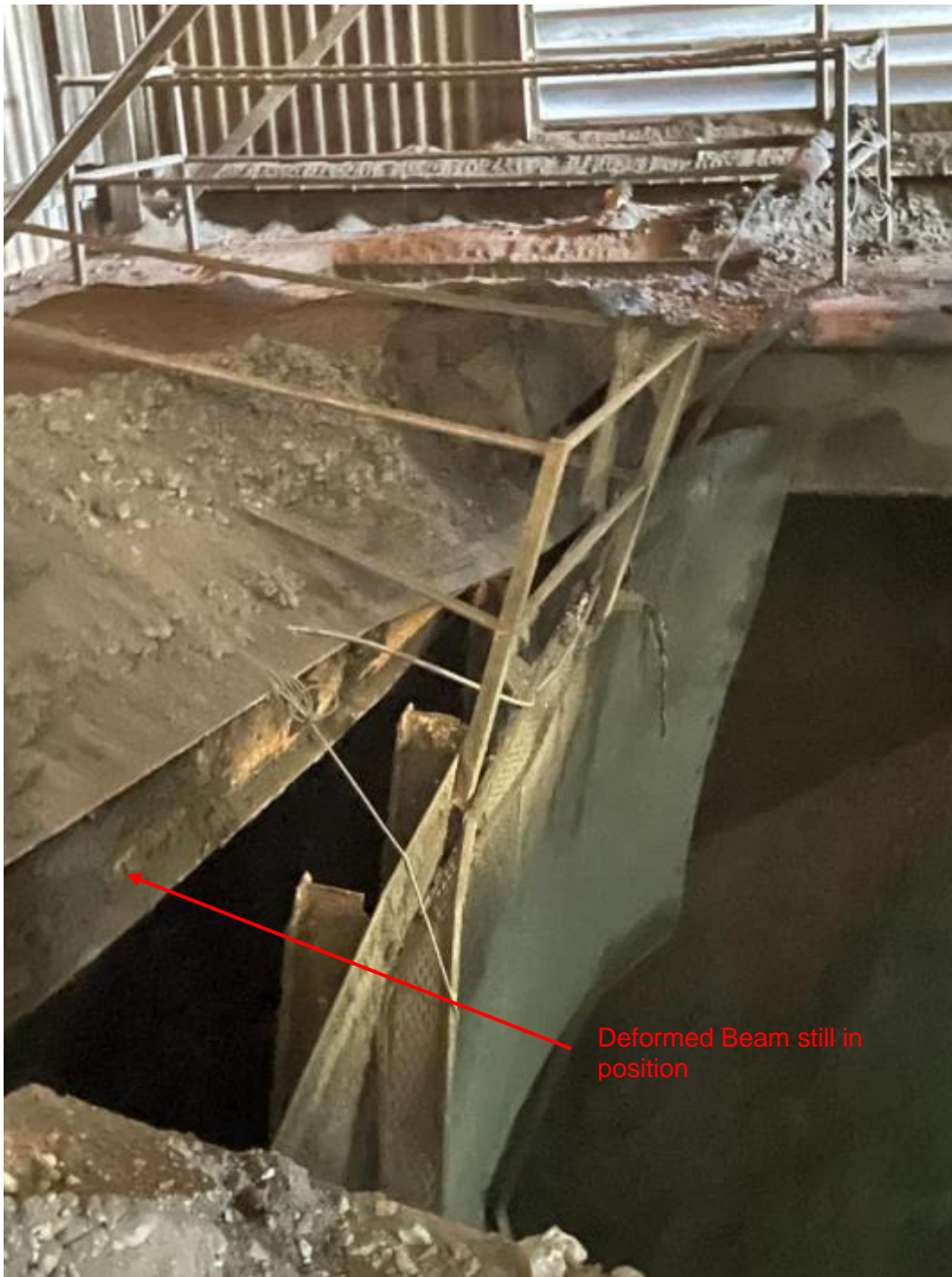
Figure 3: Deformed beam in place and section of platform removed
